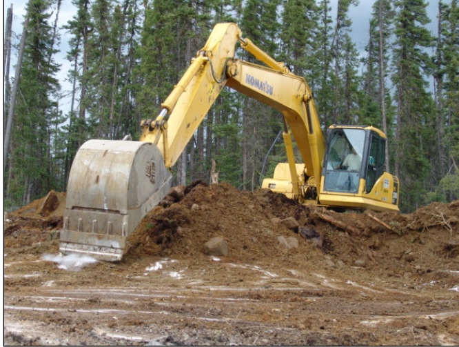
Photo 3: Backhoe being used to strip overburden.
