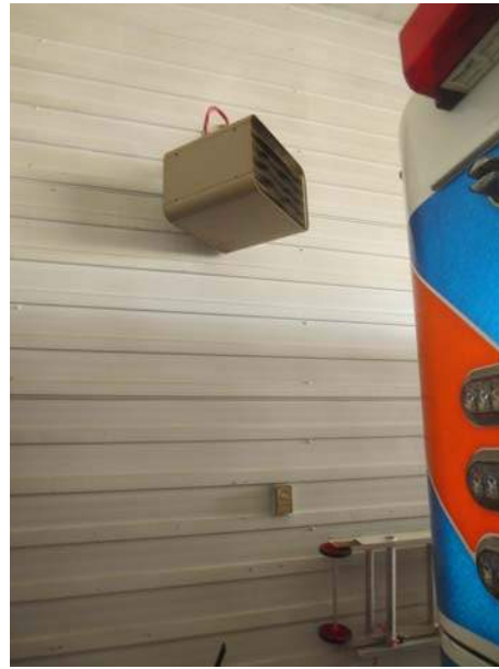
M-10 - Electric Unit Heater (Garage)
