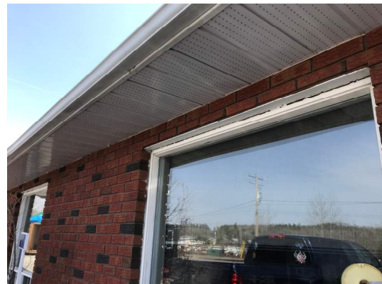
Photo 16 – Wood/Vinyl windows in poor condition and sealant failure
