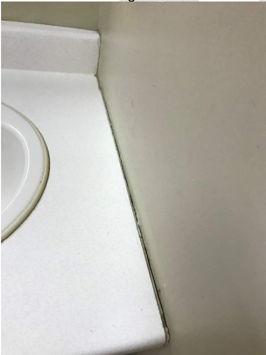
Photo 30 – Seals missing at washroom counters
