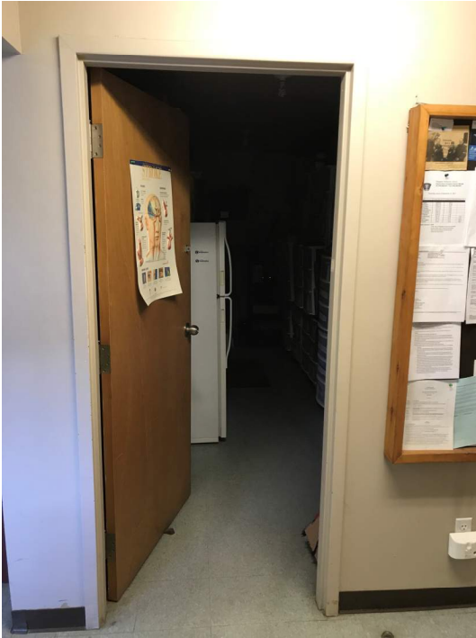
Photo 25 – Typical wood door with knob style hardware, chips in hollow metal frame paint finish.
