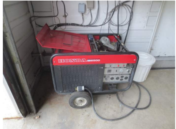
E-8 - Emergency Generator (Honda 6.5 kW)
