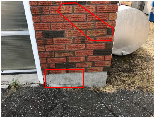
Photo 11 – Step cracking at SW corner
