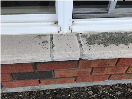
Photo 12 – Cracked mortar at concrete copings
