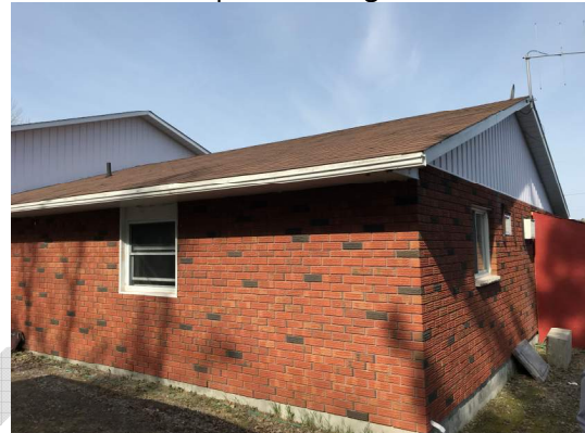
Photo 14 – No drip edge or venting of roofs. No apparent metal flashing at vinyl siding to upper roof Downspouts missing or disconnected.
