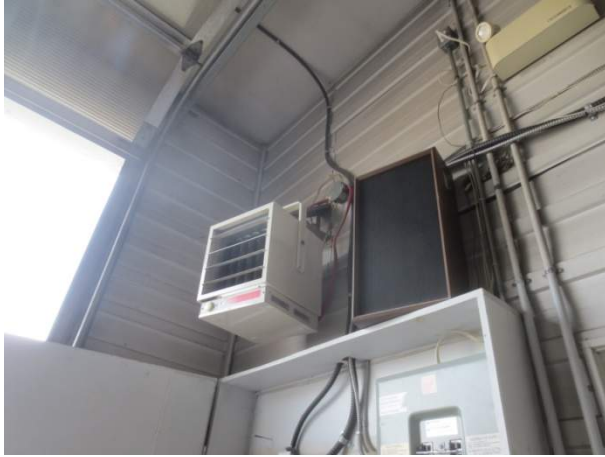
M-9- Electric Unit Heater (Garage)
