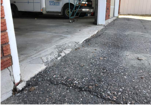
Photo 21 – O/H door rusting frames and chipped sills/foundations
