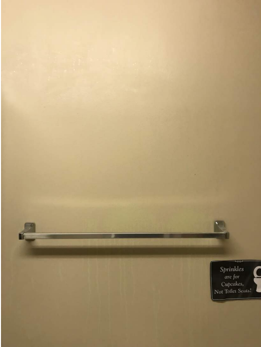
Photo 29 – Moisture streaks in paint in washrooms.
