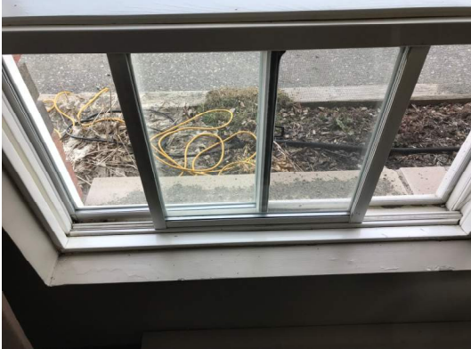
Photo 17 – Window weather-stripping broken. Sealants have failed.
