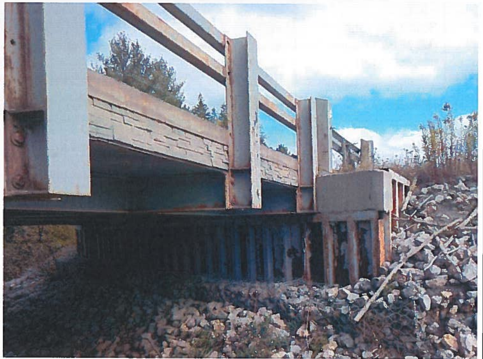
Photo 4: SE Corner of Bridge – note wide crack in concrete ballast wall and broken approach guide rail post.
