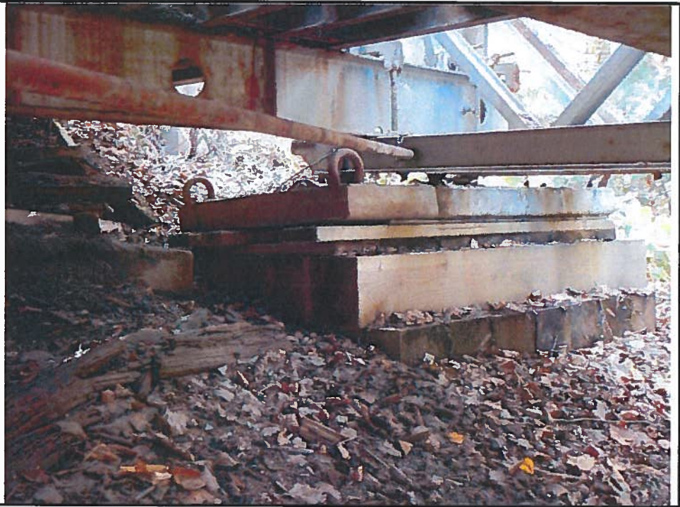
Photo 5: Settlement at SW Bearing (Similar SE and NE Bearing)
