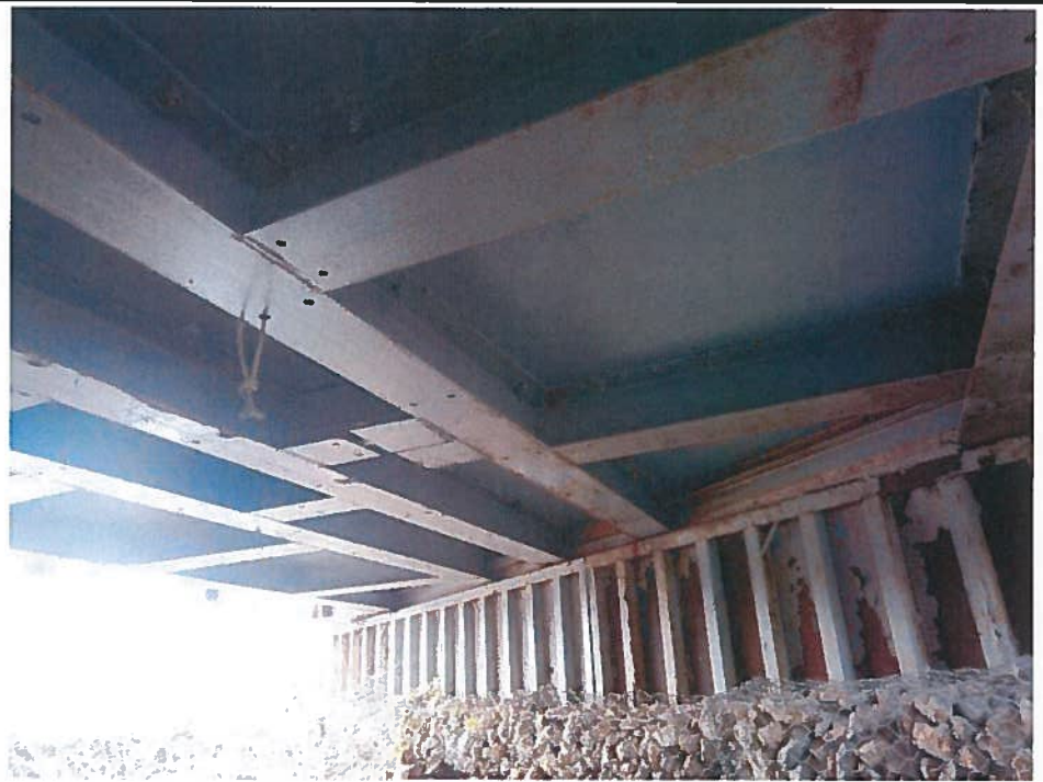
Photo 5: Bridge Soffit – showing deck panel link member
