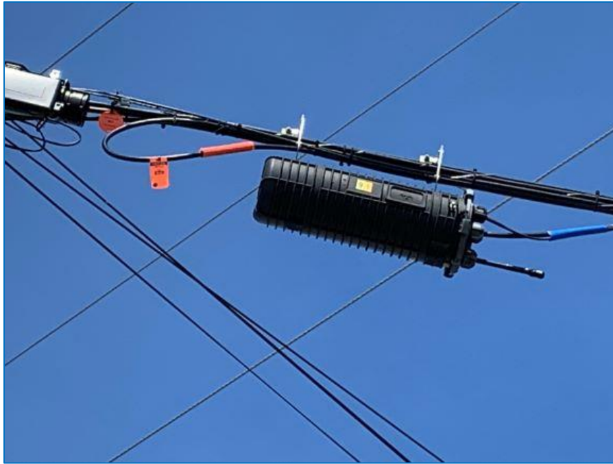
Figure 40: Ontera aerial fibre tag
