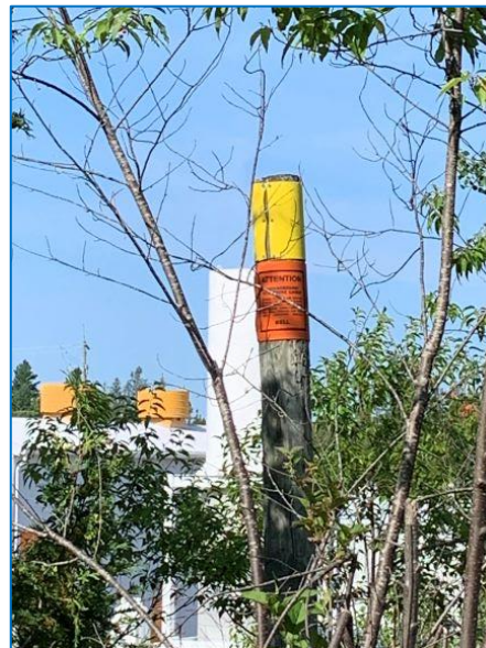
Figure 47: Bell buried fibre marker
