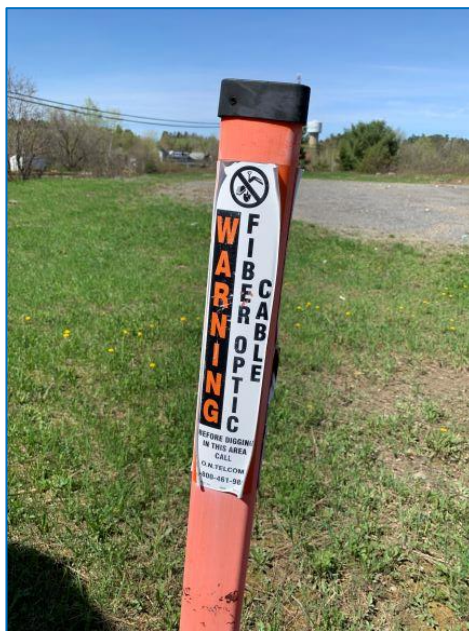
Figure 41: Ontera buried fibre marker
