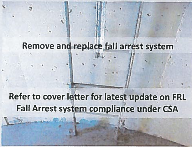
Anti-slip tape required on smooth ladder rungs
