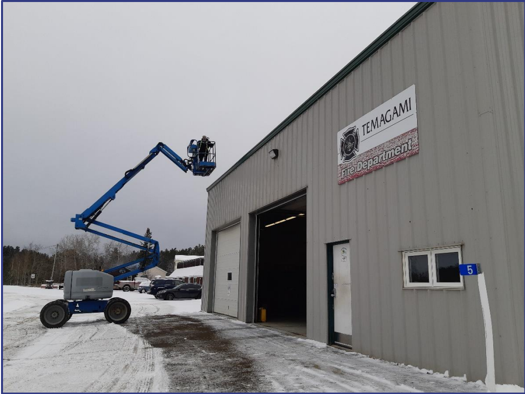
Photograph 1: West elevation of building
