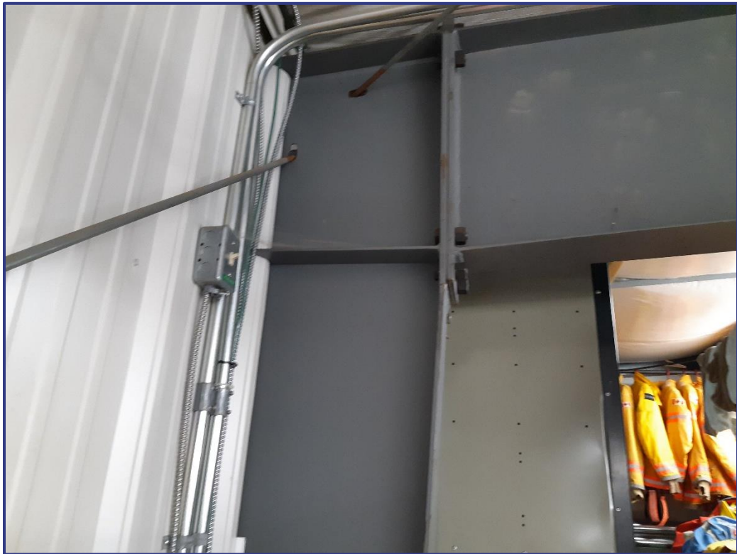
Photograph 4: View of main steel frame
