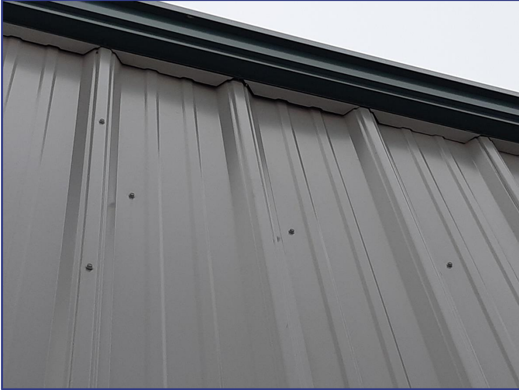
Photograph 11: General view of building sidewall with flashing
