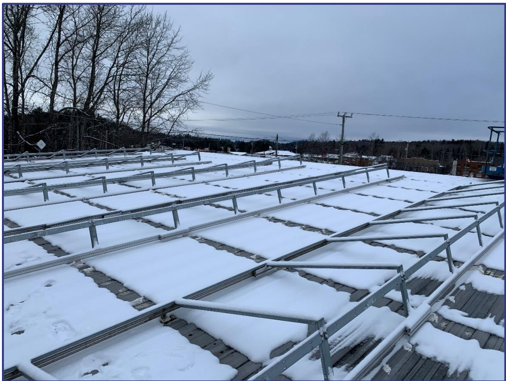
Photograph 2: General view of roof with solar panel brackets
