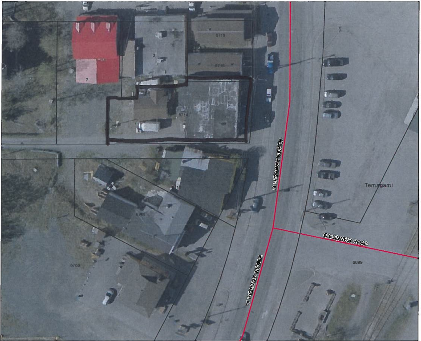
P4 6714 Hwy 11 north the Spooner Building
