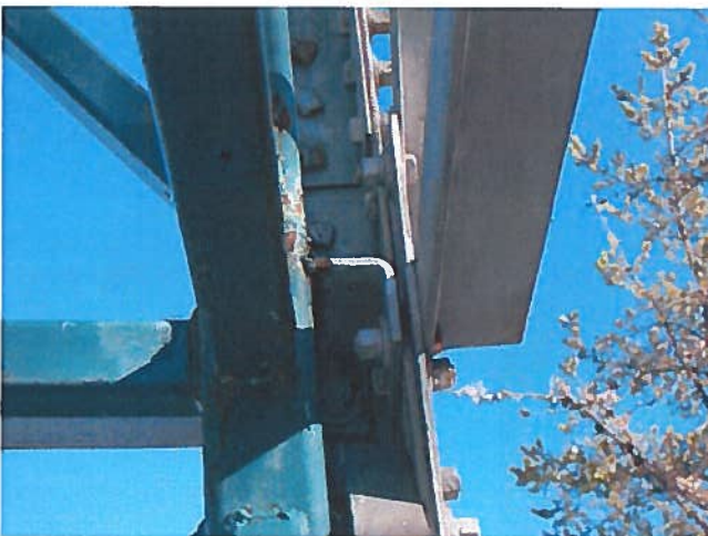
Example of installed weep hole
