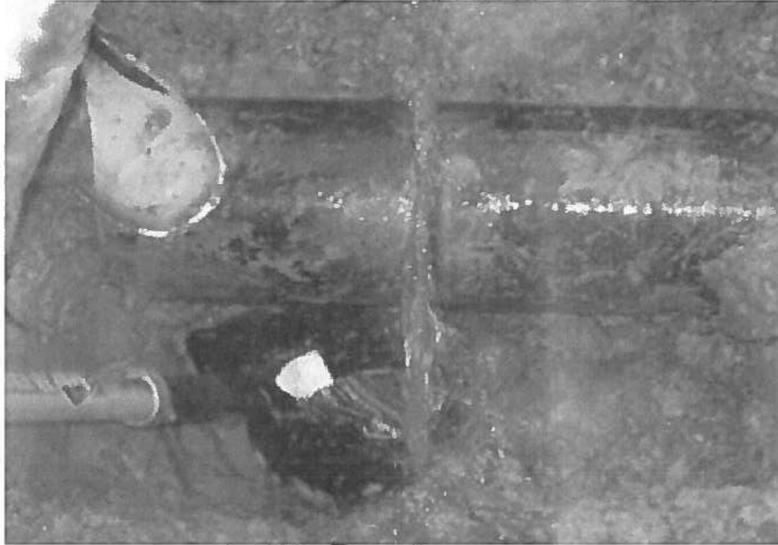
Figure C-1: Circumferential watermain break with flow maintained until after an Air Gap was created.
