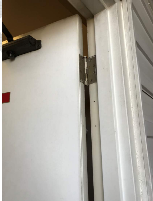
Photo 32 – Rating label missing on interior door from garage to vestibule
