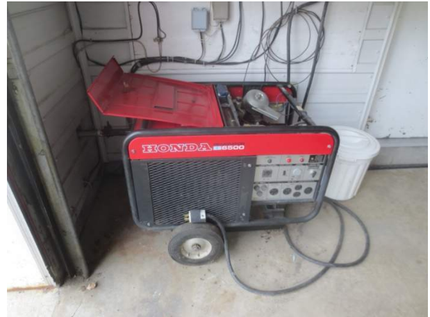
E-8 - Emergency Generator (Honda 6.5 kW)
