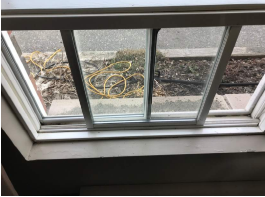
Photo 17 – Window weather-stripping broken. Sealants have failed.
