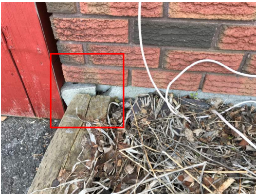
Photo 8 – Spalling of parging and block S-E corner
