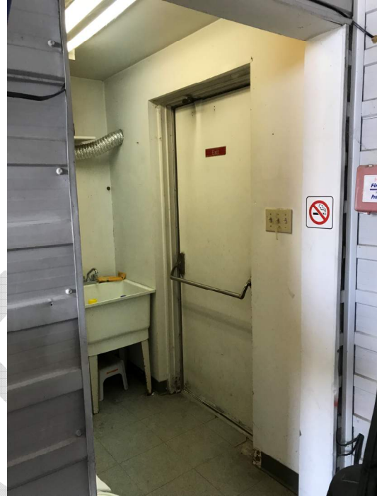
Photo 19 – Exit/service door rust and missing hardware
