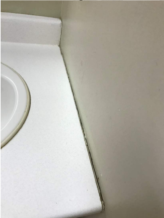
Photo 30 – Seals missing at washroom counters
