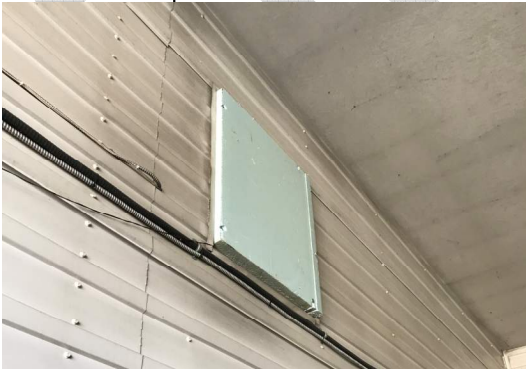
Photo 35 - Access panel not rated closure and covered with exposed foam insulation
