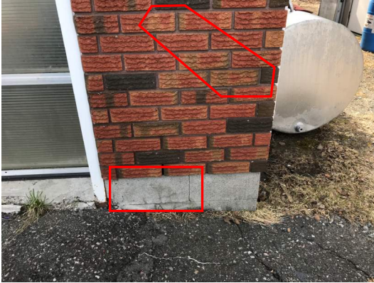
Photo 11 – Step cracking at SW corner
