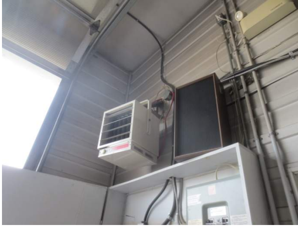
M-9- Electric Unit Heater (Garage)
