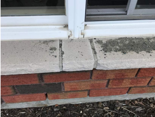
Photo 12 – Cracked mortar at concrete copings
