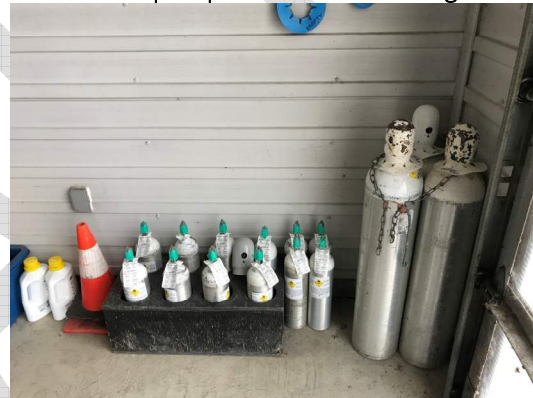
Photo 37 – Oxygen tank storage. Some tanks loose and require protection from damage.
