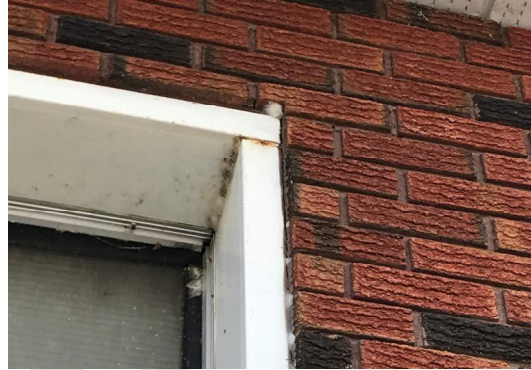
Photo 22 – O/H door lintel to be confirmed. Weather stripping and sealant deteriorating.
