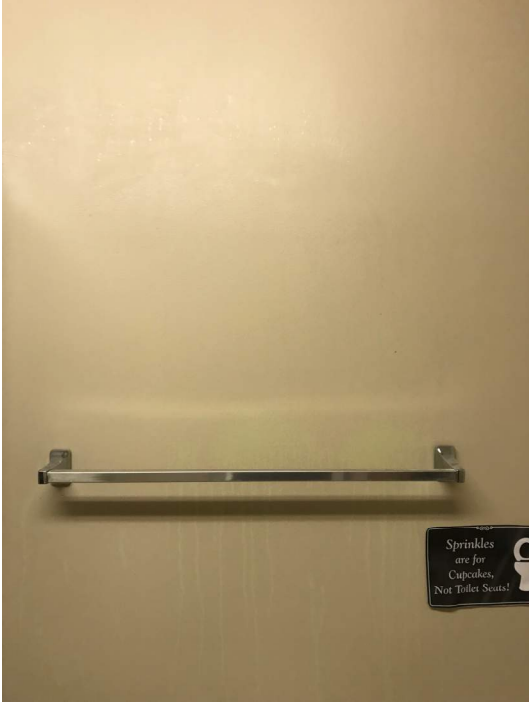
Photo 29 – Moisture streaks in paint in washrooms.
