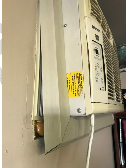
Photo 24 – Gaps at thru-wall A/C units
