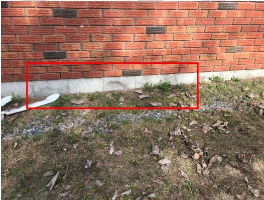
Photo 8 – Spalling of parging and block S-E corner
