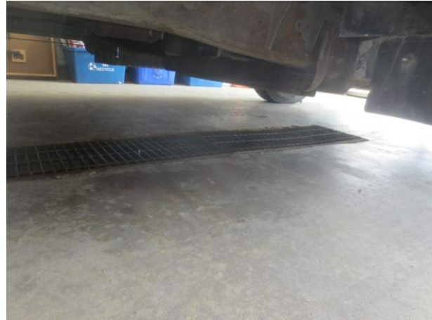
M-6 - Trench Drains (Garage)
