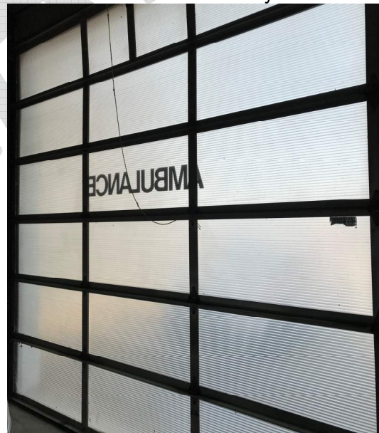
Photo 20 – O/H door not thermally insulated
