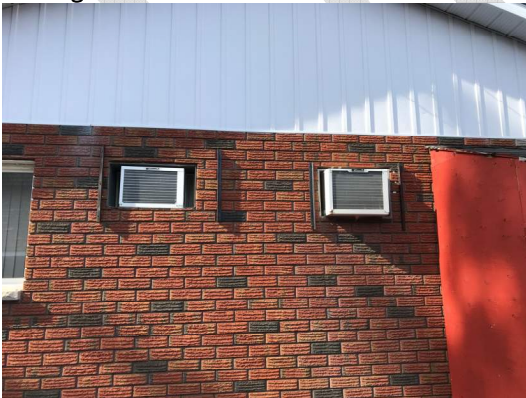
Photo 13 – Caulking of Vinyl and Drip trim missing
