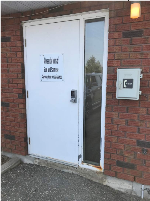
Photo 18 – Entrance Door rusting frame and Non barrier free accessible step.
