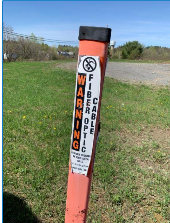
Figure 44: Ontera buried fibre marker
