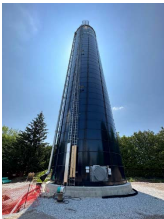
Photo 1: New GFS Port Lambton Standpipe
