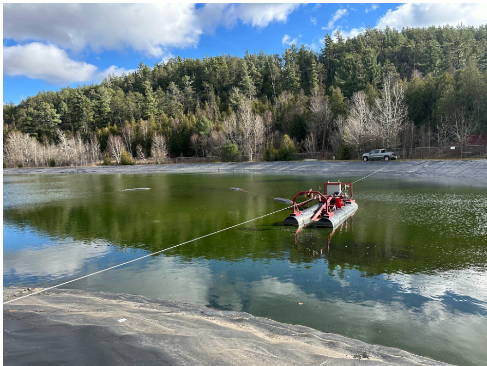
Figure 5. Dredge deployed into the lagoon cell.
