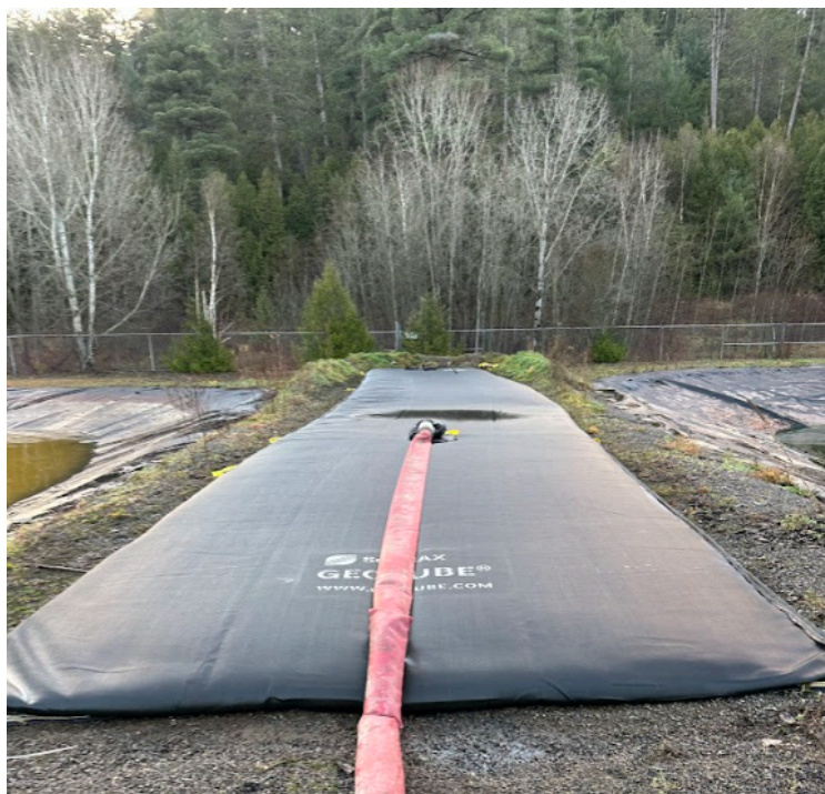
Figure 2. View of the Geotube unit onsite.
