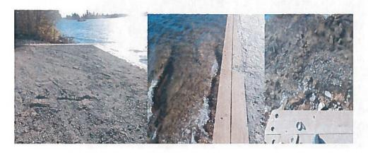
Unfortunately the far end of new dock ramp area is very shallow and not useable as a loading area. It is being recommended that one row of four older docks be attached and added off this area. About 18-20 feet in from the far end of the Wall. Contractors could then approach both sides of this dock area pointing in and could load off their front of their boats. The farther area along the docks could be also be used as a loading or unloading area or for short term docking.
