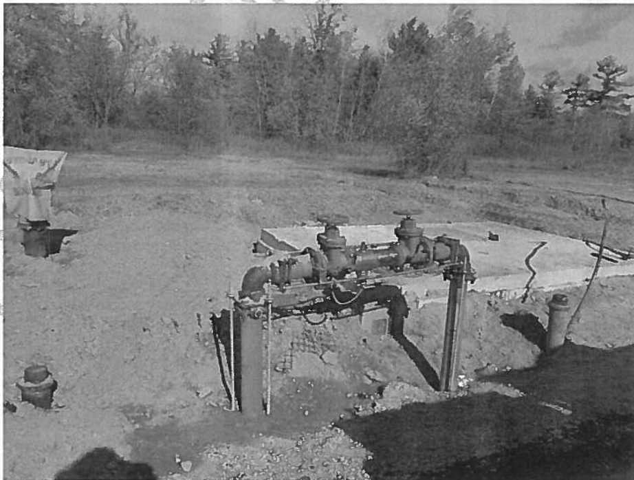
Figure A-2: Temporary connection from watermain with Backflow Prevention with a CSA approved reduced pressure backflow preventer
